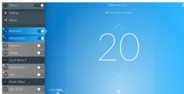
Indoor Unit Activated
